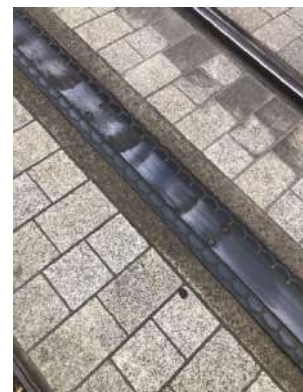
This photo shows the scuff marks on the centre rail made from the skate.
