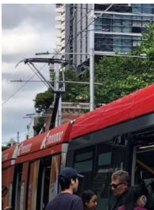
This photo shows the pantograph up and contacting the catenary as it stops at City Hall.
